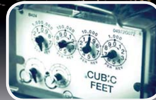
Gas & Water Metering
